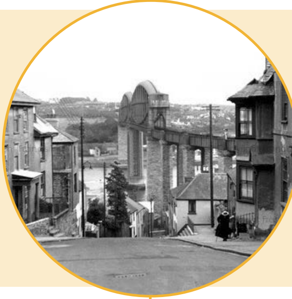
Picture of the Royal Albert Bridge from Lower Fore Street in 1955.
