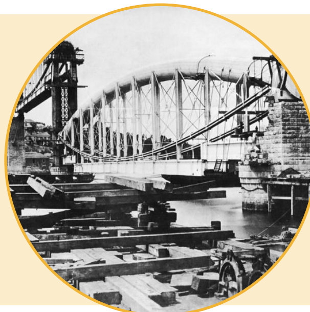
The Royal Albert Bridge during constructions in the 1850's. The bridge has been open since May 1859 and is a major attraction of Cornwall and the Southwest.
