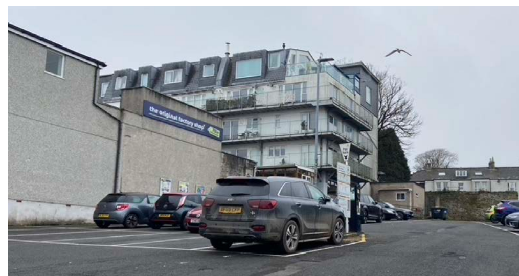
Belle Vue Carpark West
